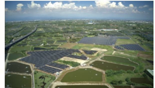
Ground type and UHV field, Beimen, Tainan
